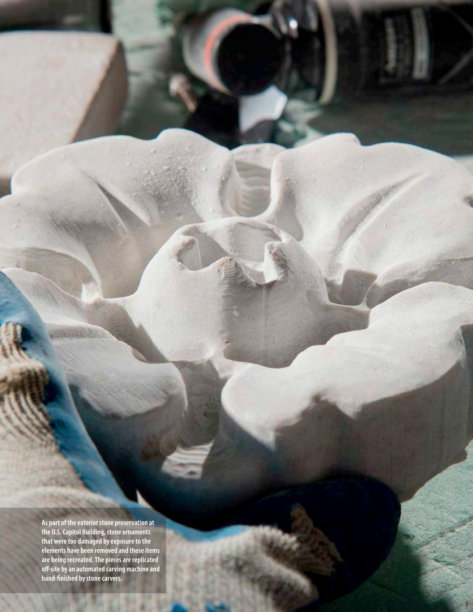
As part of the exterior stone preservation at the U.S. Capitol Building, stone ornaments that were too damaged by exposure to the elements have been removed and those items are being recreated. The pieces are replicated off-site by an automated carving machine and hand-finished by stone carvers.
