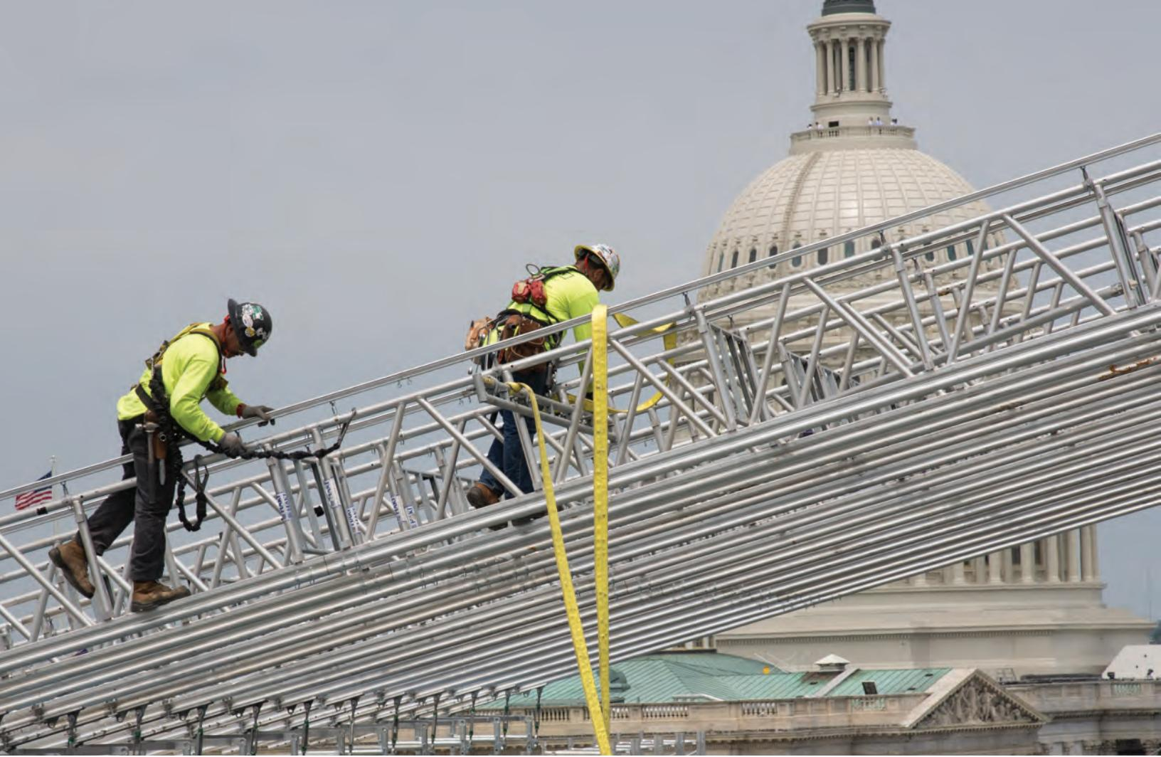
As part of the Cannon Renewal Project, the AOC erected a protective roof covering system on the Cannon Building's west wing. The temporary system will surround the existing roof during the demolition of the facility's fifth floor.
