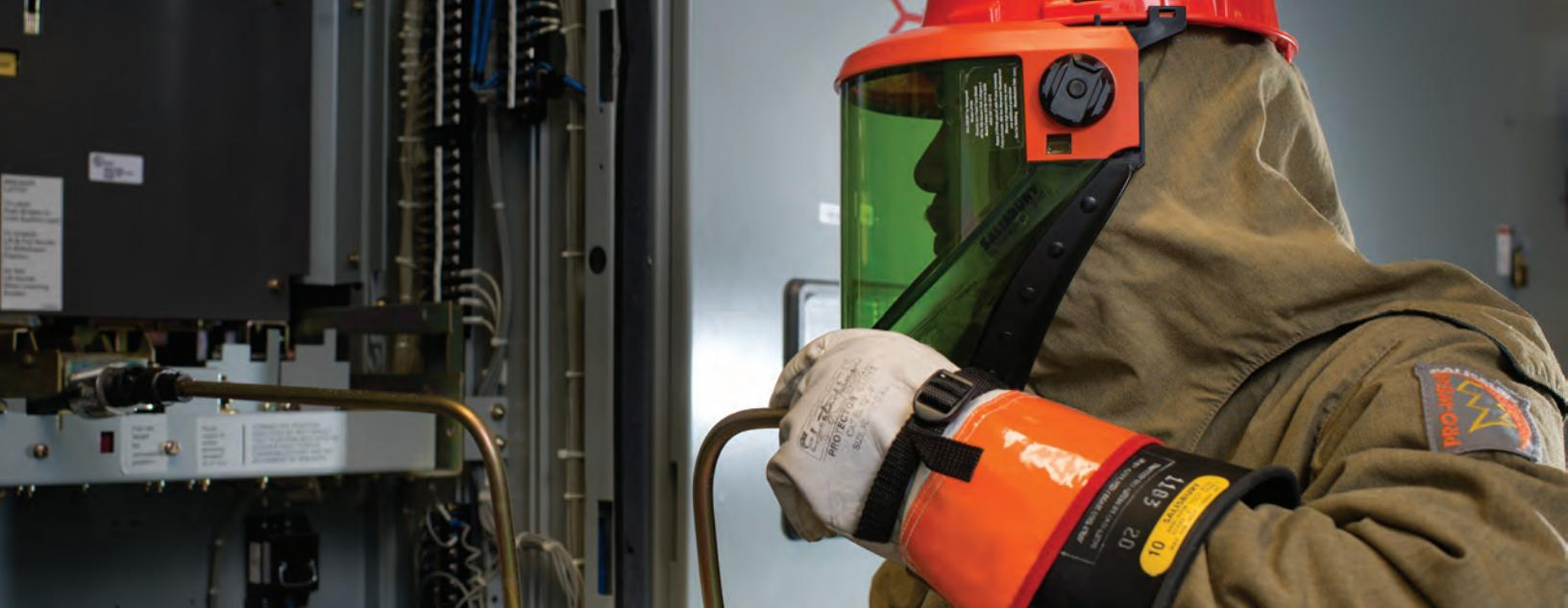
A high-voltage electrician follows precise procedures and wears a fireproof suit while performing routine preventative maintenance on a 15,000 volt circuit. Safety training and procedures are essential to the maintenance of industrial equipment and systems at the AOC.
