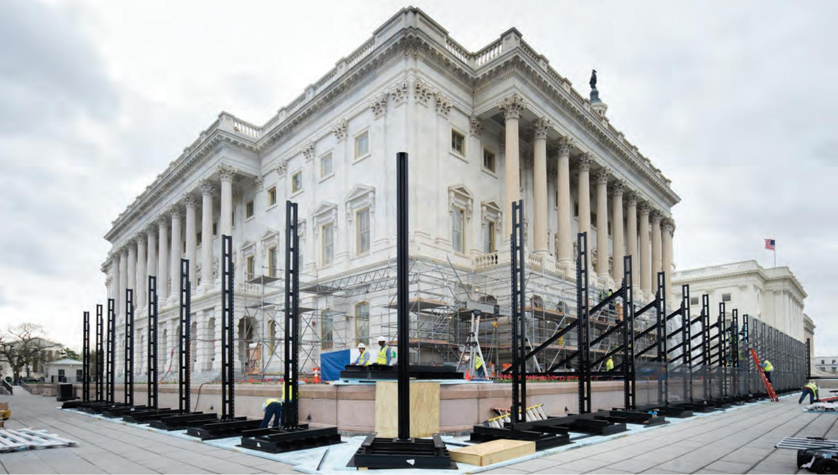
The U.S. Capitol Exterior Stone and Metal Preservation Project is a multi-phased project designed to address deferred maintenance, extend the life expectancy of the deteriorated stone and replace missing elements of the U.S. Capitol Building.
