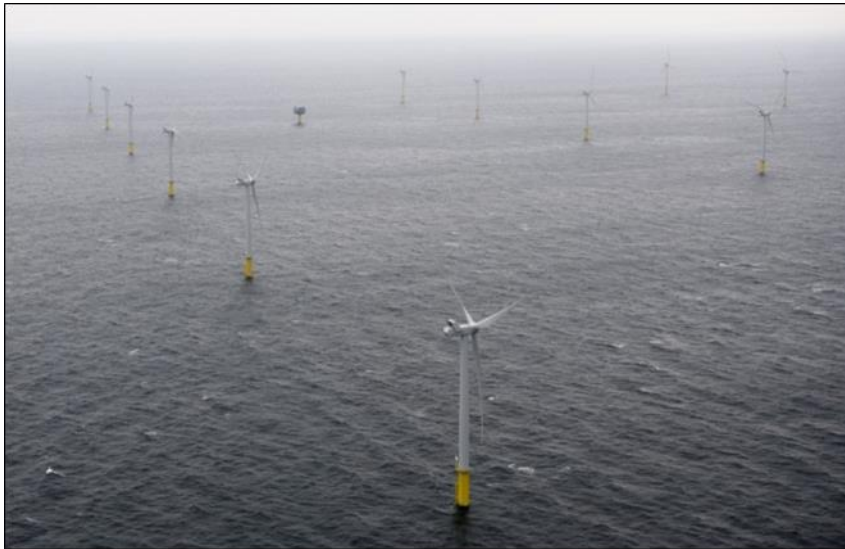
Figure 7-2 Monopiles with wind turbines (OWF Luchterduinen)
