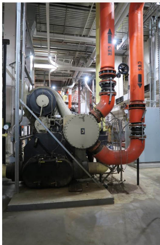
Figure 68. Existing Chiller (#3)
