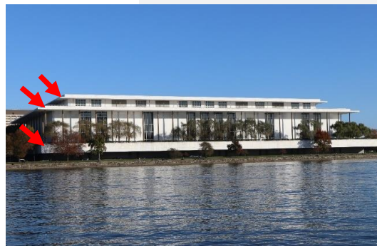
Figure 1. The Kennedy Center Rock Creek Parkway (lowest arrow), Plaza Level (middle arrow), and Terrace Level (uppermost arrow) overhangs (west facade shown).
