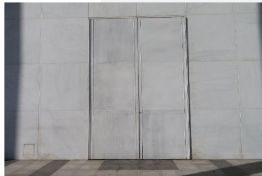
Figure 24. Plaza Level east facade load-in doors with faux marble finish.
