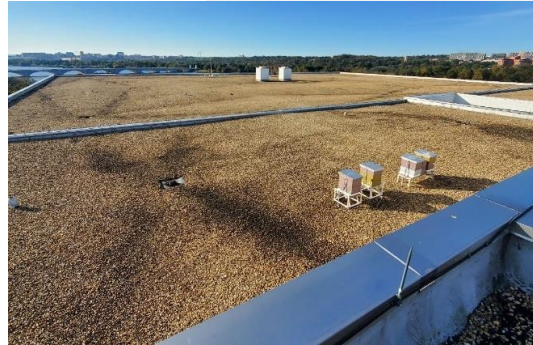
Figure 38. Main Roof gravel-surfaced coal tar pitch BUR roof membrane assembly with stainless steel coping and counterflashing's.
