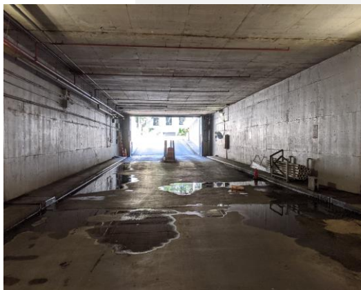
Figure 61. Service Tunnel Entrance
