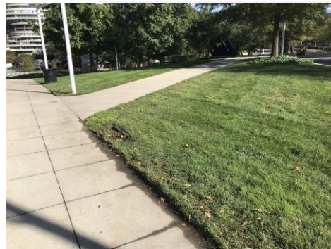
Figure 83. Concrete Sidewalk and Lawn Area
