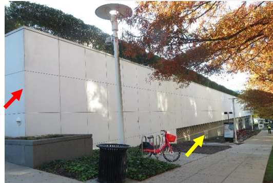
Figure 14. Cast-in-place concrete (yellow arrow) and precast concrete panel (red arrow) exterior walls at the north facade.
