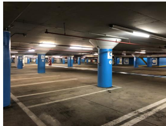
Figure 87. Parking Garage Level C
