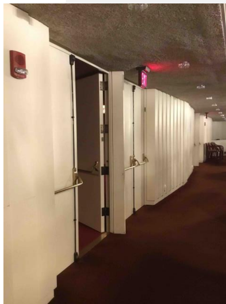
Figure 63. Acoustical Door at Theater Entrance
